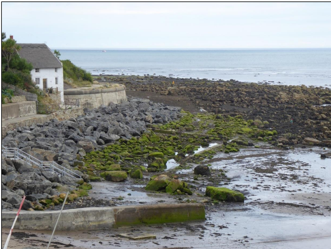
Figure 2.1. Location of new granite rock armour at the foot of the seawall, note the green (colonised) natural boulders which have been placed in front of the granite rock (August 2018).
